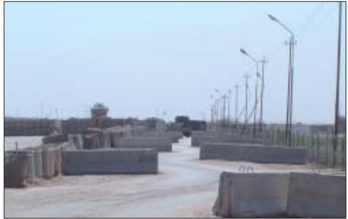
Entry Control Points with only one lane of traffic and sufficient obstacles to deny high speed-access offered the best defense against vehicle-borne improvised explosive devices and suicide bombers.
