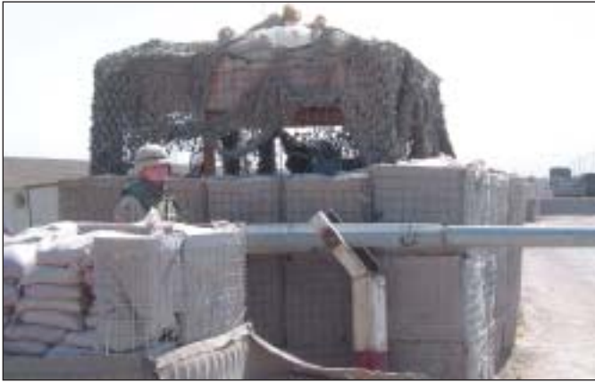
Entry Control Points with only one lane of traffic and sufficient obstacles to deny high speed-access offered the best defense against vehicle-borne improvised explosive devices and suicide bombers.
